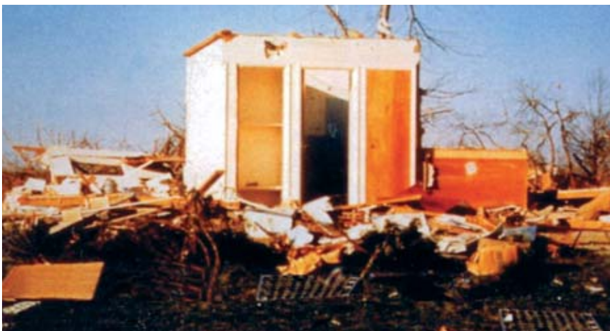
This interior room remains standing after a storm.
