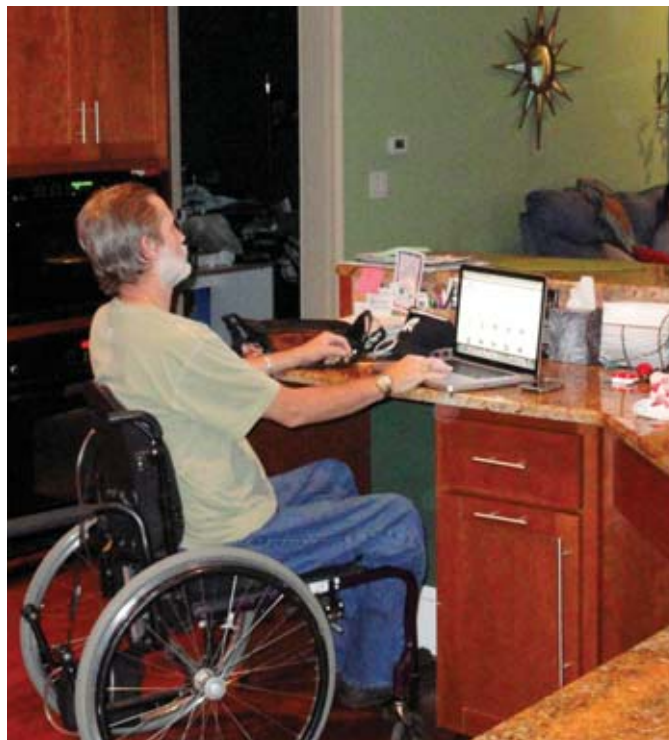
A full office is not always needed. Here, John has removed the rolling cart under the kitchen-sink island and uses this space for computer work and as a play station. This allows him to hang out with the rest of the family and use his computer because knee space was provided.
